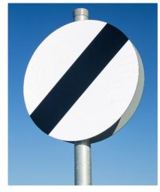
Aluminium sheet metal road sign bolted to a galvanised steel post
